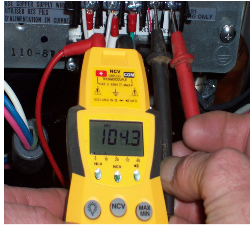
Outdoor unit at U1 & U2 communication line
